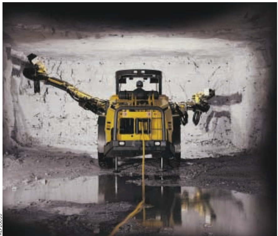
An Atlas Copco drilling rig at work in a Swedish tunneling project, equipped with a Cavotec Specimas cable reel and Cavotec Connectors.
