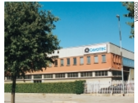
Cavotec Specimas manufacturing facility near Milan.
