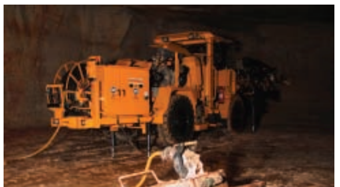
Cavotec reel and connector at work on a drilling rig, Sweden
